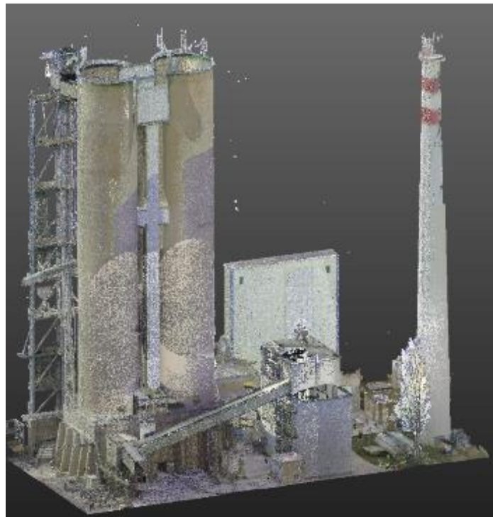
Fig. 6. Georeferenced TLS point cloud of the investigated homogenization silos
