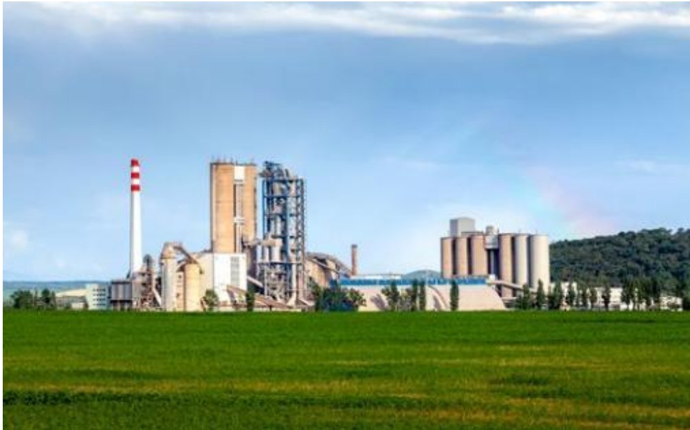
Fig. 1. View of the cement plant and the object of research
